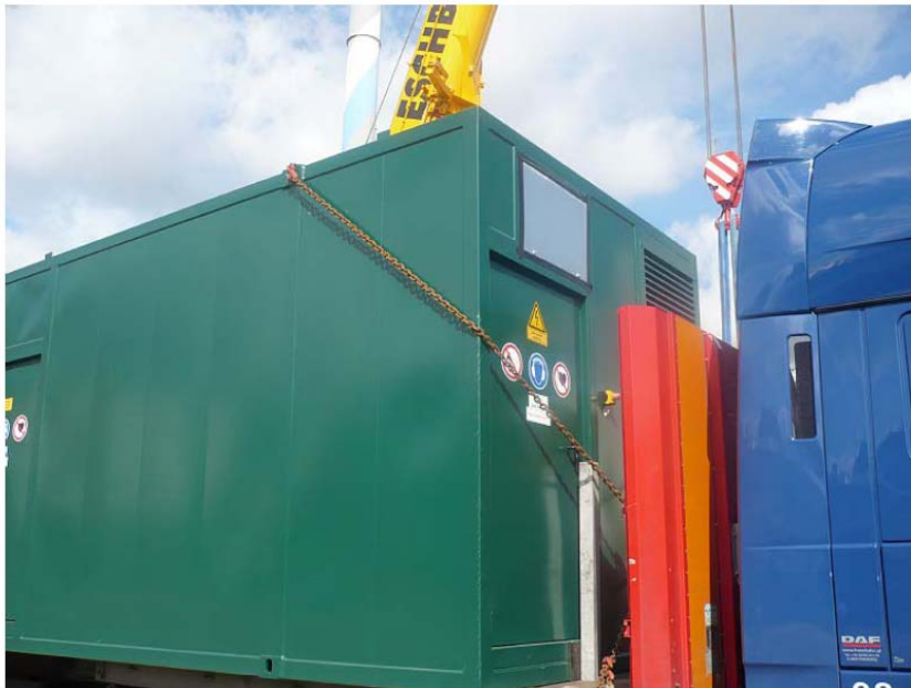
Fig. 18.15 This fastening leads to dents and paint damage on the container
